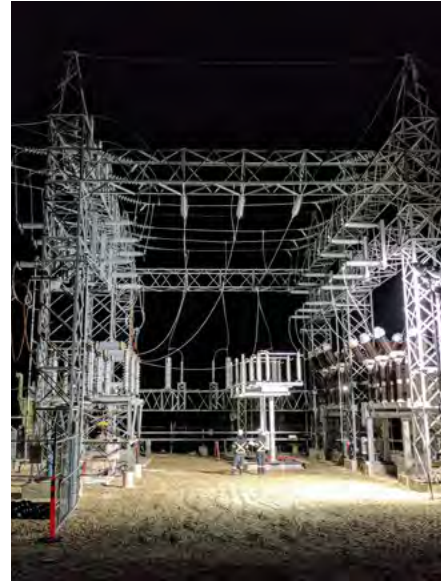
3 NEW SUBSTATIONS CONSTRUCTED
