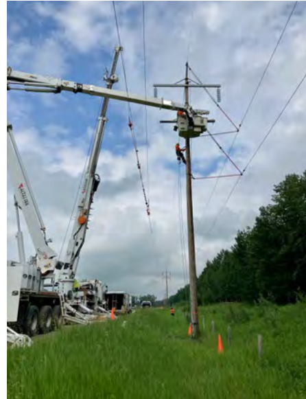
300 KILOMETRES OF NEW TRANSMISSION LINE INSTALLED
